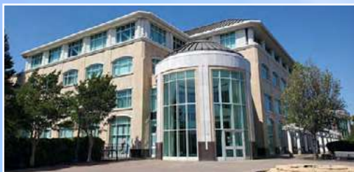
John O'Lague Galleria at Hayward City Hall 777 B St, Hayward City Hall, Hayward, CA 94541 www.haywardartscouncil.org
